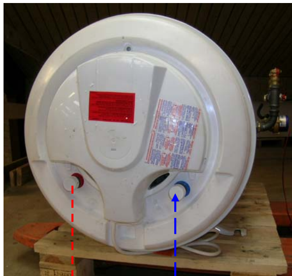
Pre-heated water out Cold water in
